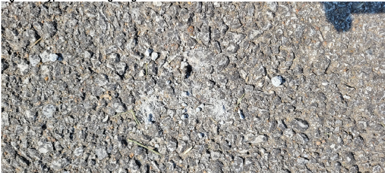
Figure 1: Typical Raveling Image
