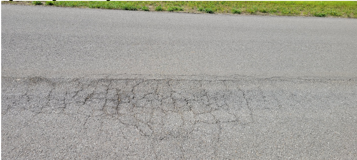
Figure 3: Alligator Cracking
